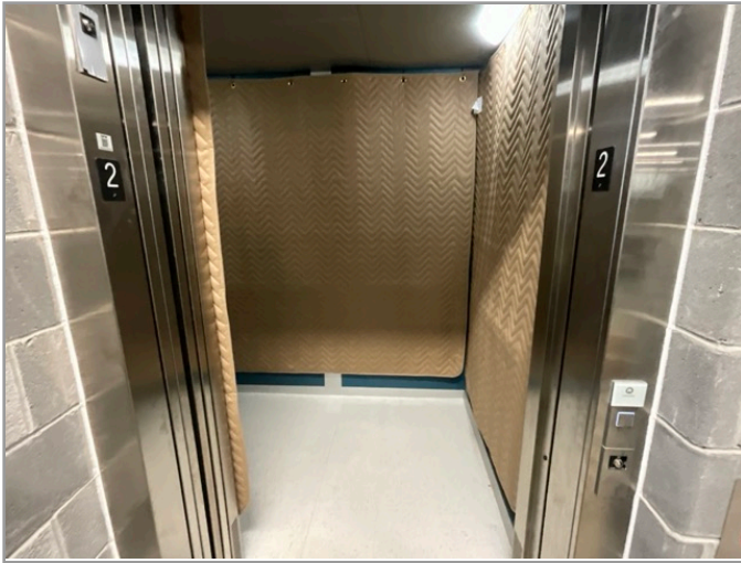
LOBBY LOOKING AT CABS (WITH DOORS OPEN)
