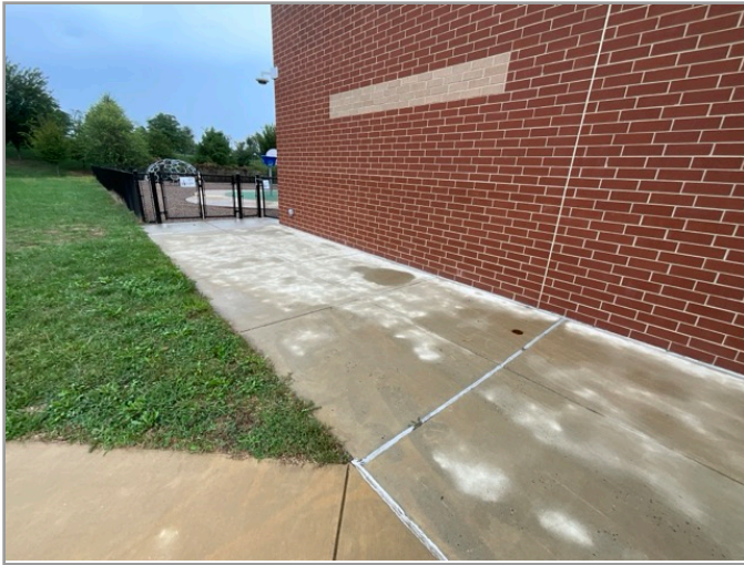
ACCESSIBLE ROUTE TO PLAYGROUND
